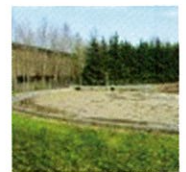
Waste Water Treatment Plant
